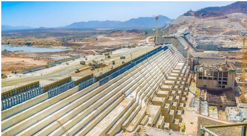
Figure 8.8 GERD (Grand Ethiopian Renaissance Dam) construction
