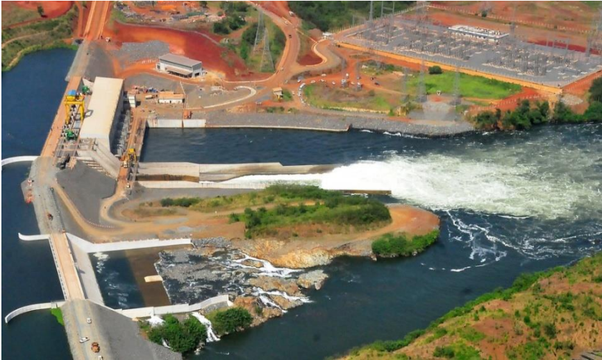
Figure 8.9 Bujagali Power Station in Uganda
