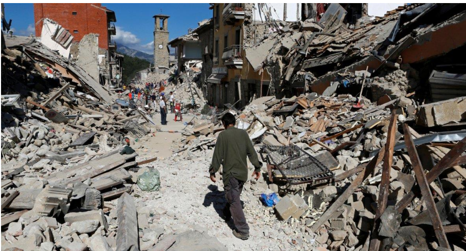
Figure 2.1 buildings destroyed by an Earthquake in Italy.
