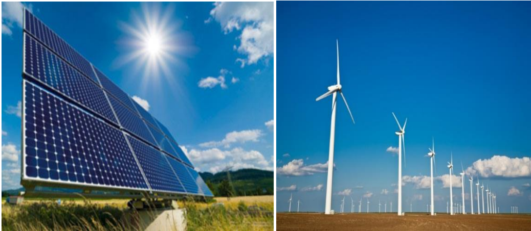
Figure 6.1 solar and wind energy power.
