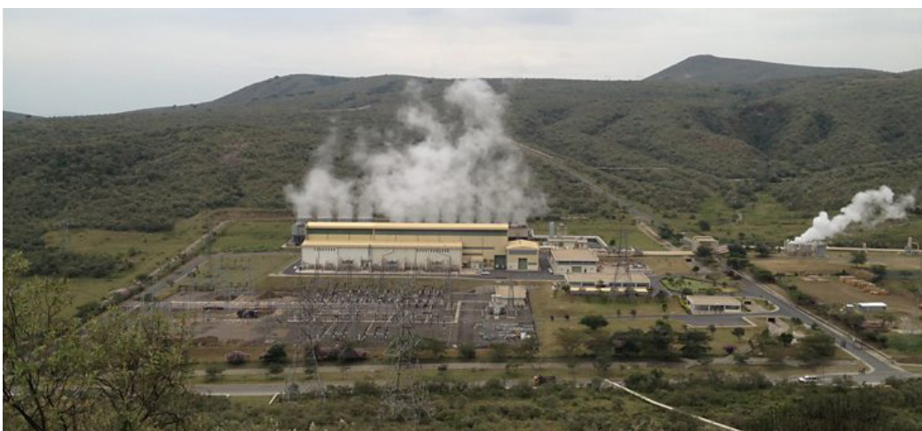
Fig. 5.16 Geothermal power station
