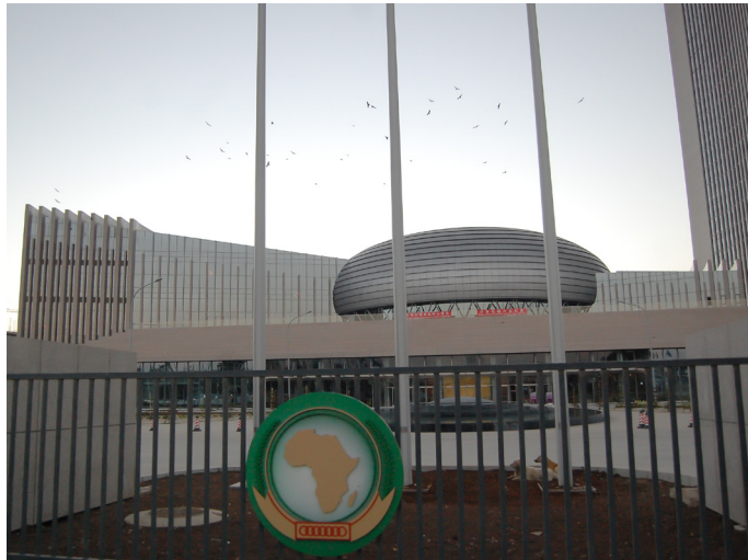
Fig. 7.4: African Union Conference Centre in Addis Ababa
