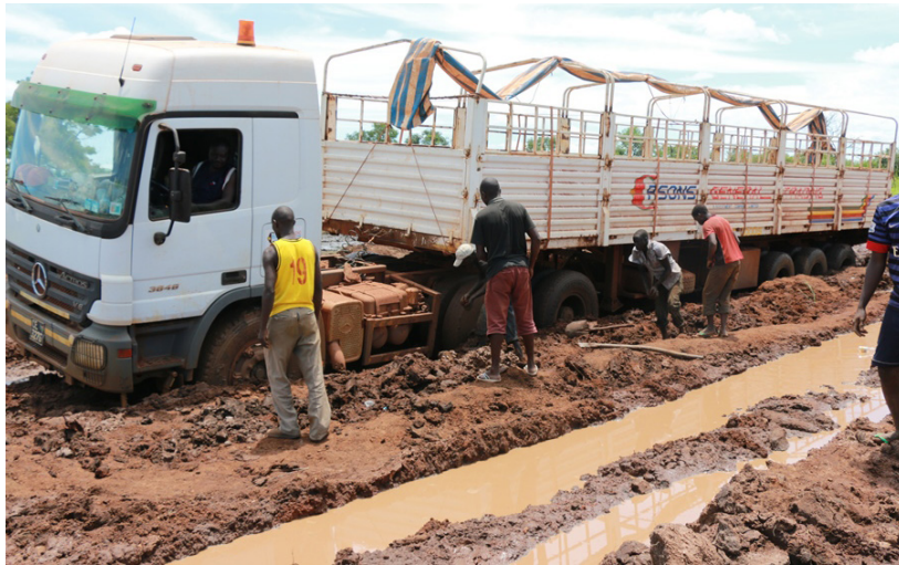
Fig. 7.8: Poor road infrastructure
