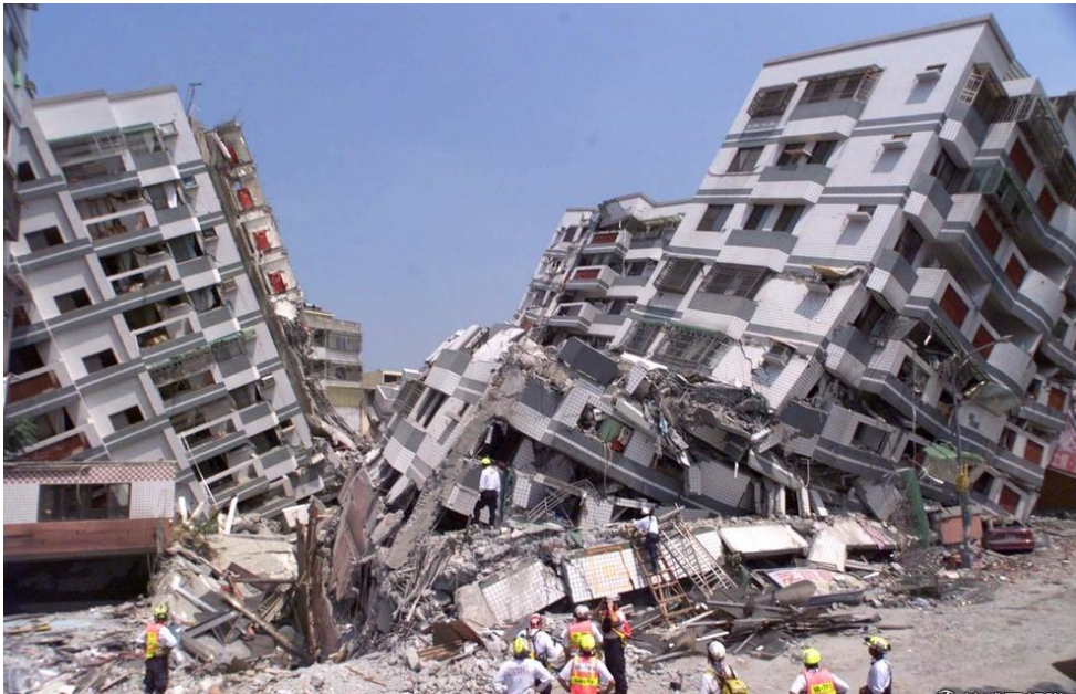
Figure 3.7 a collapsed building due to an earthquake in Japan.
