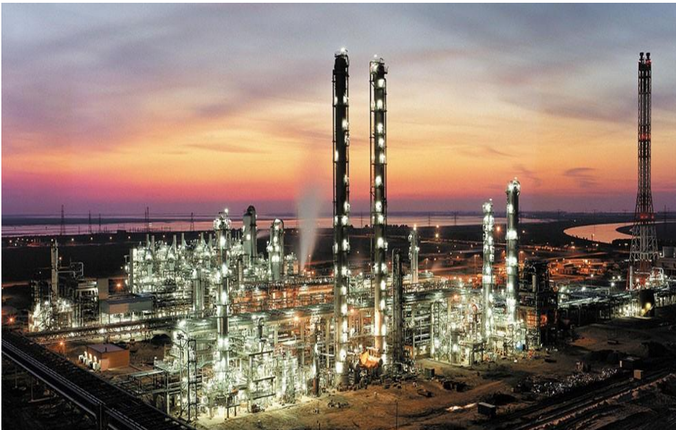
Figure 7.3 an oil and gas company in South East Asia.
