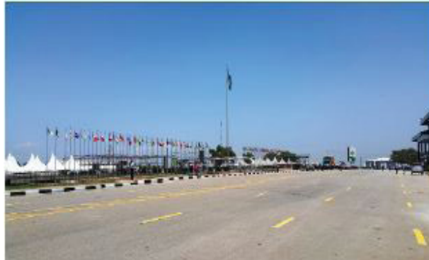
Construction of new roads
