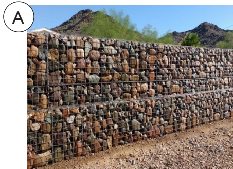
Building of check dams or gabions.
