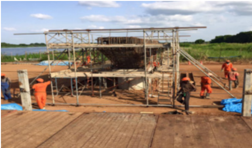
People building a bridge
